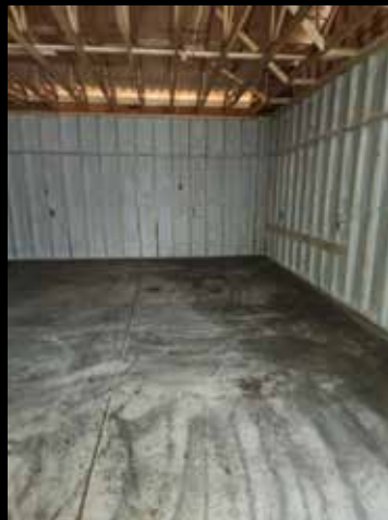
Spray foam insulation was added to the new addition and also all exterior walls on the existing building to be a little more energy efficient over the existing exposed brick.
