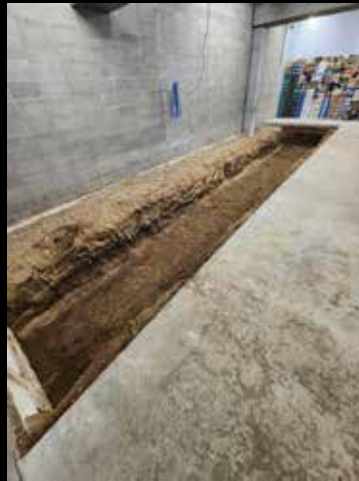
The existing backroom/warehouse was prepared for footings and a ramp to be built for access between two buildings
